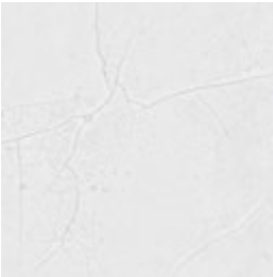
Cracked white 20MM
